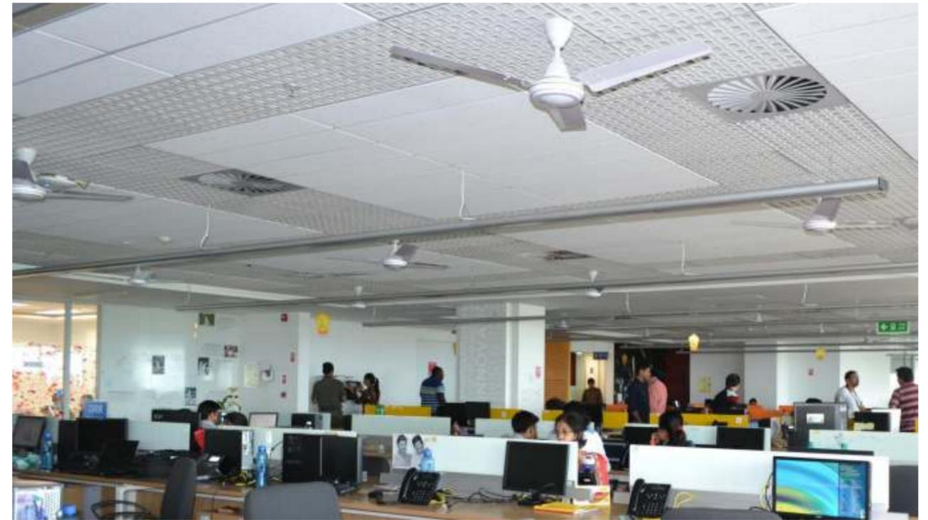
▲ In India, facilities have started providing ceiling fans in mechanically ventilated spaces to enhance the air movement. This contributes to better thermal sensation and improves performance of occupants
