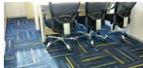
◀ Carpets eliminate floor impact sounds such as noise produced by footfalls and chairs scraped across the floor
