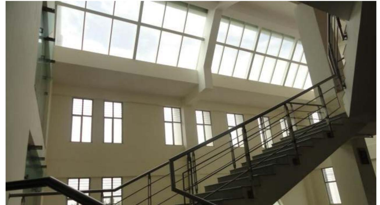
▲ Windows and skylights provided on the northern side allows maximum penetration of daylight. The north light allows maximum diffused light and minimum heat
